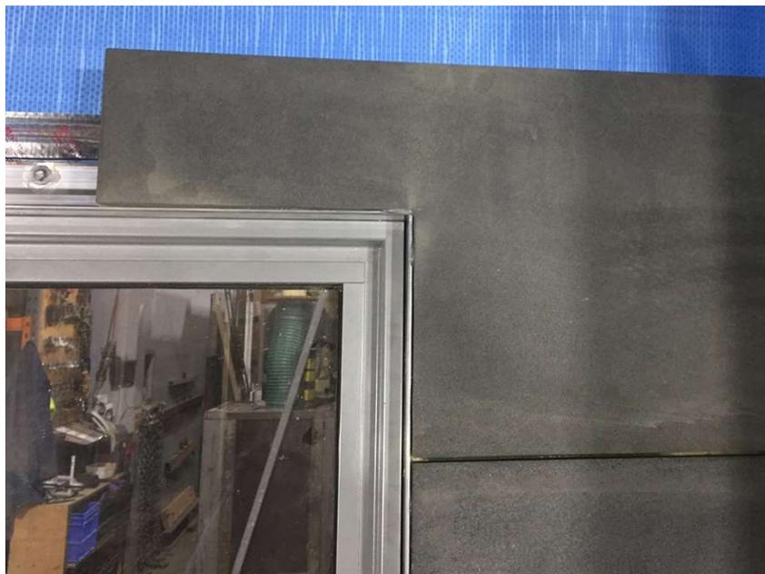
36) Should horizontal expansion joints be required or where blocks must be fitted up to an eave the clips may be used in vertical joints. At the ends short sections of wall up against block work or other adjoining cladding materials the Reveal extrusion may be cut to act as a starting clip as shown on the right in the image below.
