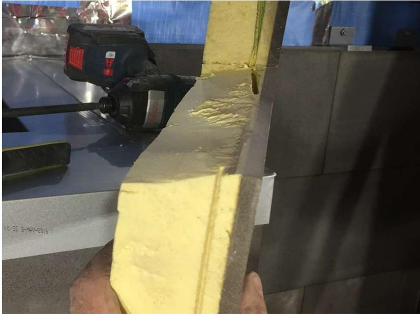
28) Tilting the top of the block forward, place the block on the locating groove below and push down to height before standing block up to ensure it is in line with the vertical wall face.
