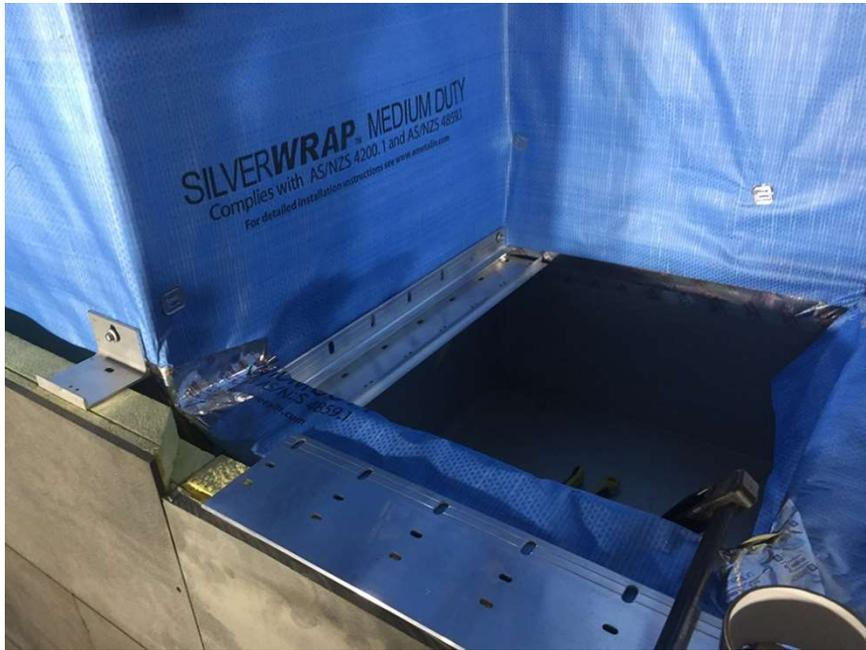
20) Flashings over parapet walls are required to ensure water tightness of the wall.
