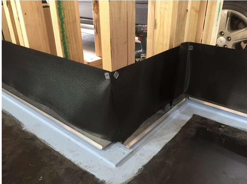
4) Sarking is then fixed to the frame according to manufacturer's directions taking care to ensure it overlaps the dampcourse by a minimum of 150mm.
