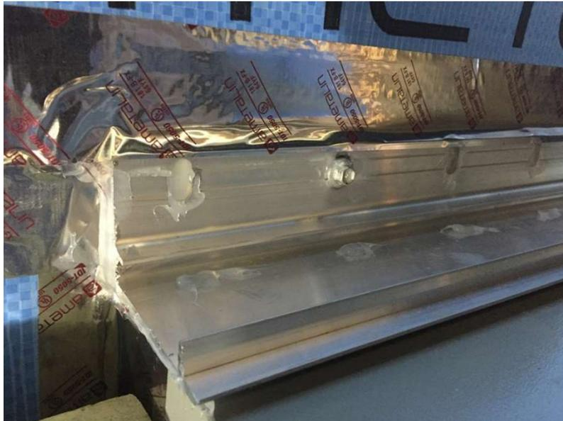
32) Blocks that are to go over the top of windows or doors must have grooves cut into them to accept the locating flanges on the Reveal extrusion both across the top and down the side of opening.
