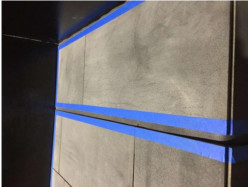
44) Sills come with a locating groove that ensures it cannot come loose once installed. The groove allows the sill to lock onto the locating flange on the Reveal extrusion. The sill may also have a 'drip-line' cut approximately 15mm back from the front edge either in the factory or done on site.
