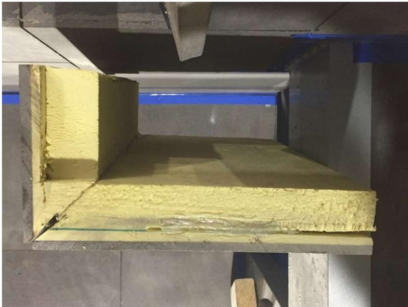
59) An 18mm thick block should be fixed to the frame and adhesive sealant applied to it and the vertical bracket flanges. The block will provide additional support to the vertical block.
