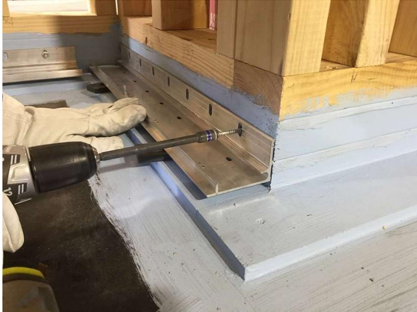
2) Care should be taken to ensure each rail is closely fitted to the next, and a maximum gap between any two extrusions of 10mm is allowed for expansion joints.
