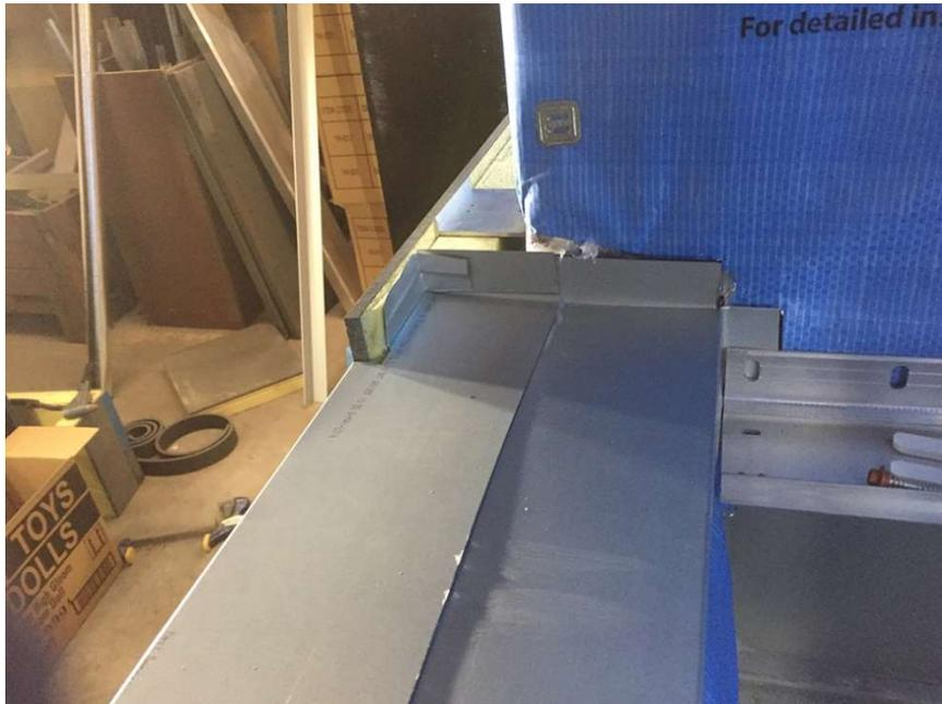
22) Flashing should be taped to sarking to ensure water tightness.
