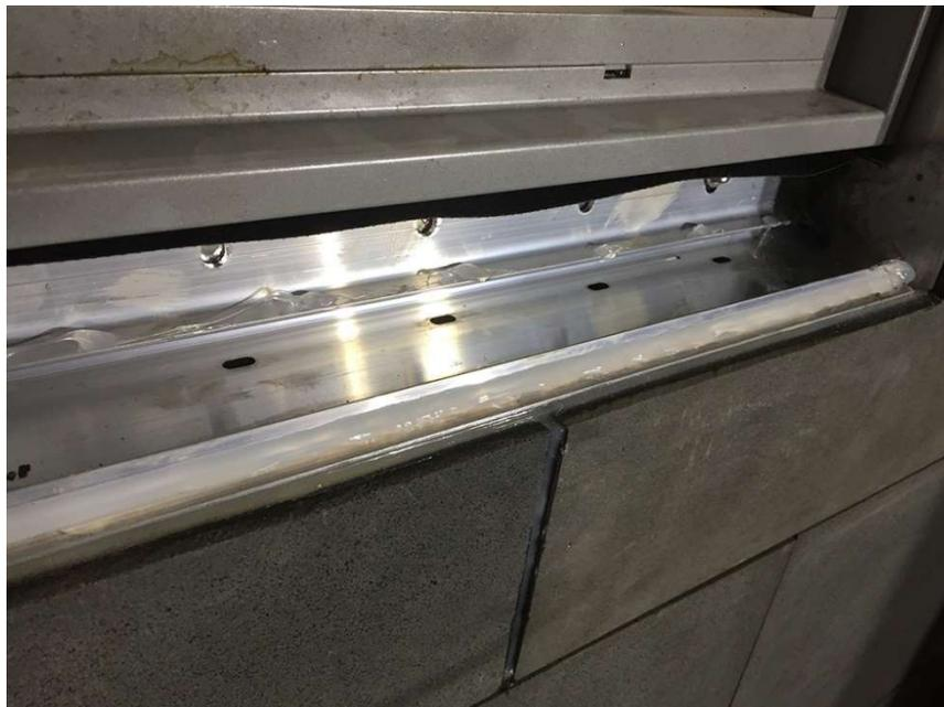
46) Place the sill below the window and lower the back edge onto the support ledge at the back of the Reveal extrusion. This will keep the back up and maintain the angle of the sill as you lower it onto the locating flange on the bottom of the Reveal extrusion.
