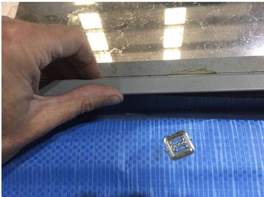
24) The Reveal Rail extrusion may be fixed below a window or door to support a SmartStone Systems sill, and may also be used vertically to close off the cavity beside the window as seen to the right of the window in the picture below.
