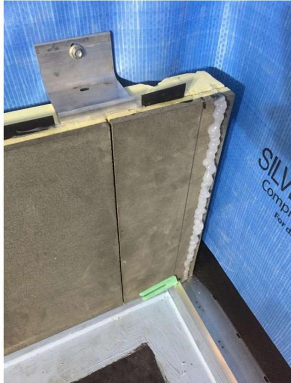
14) Where expansion joints are specified for structural purposes a 10mm gap is left that must have backing rod inserted before being filled with flexible sealant.
